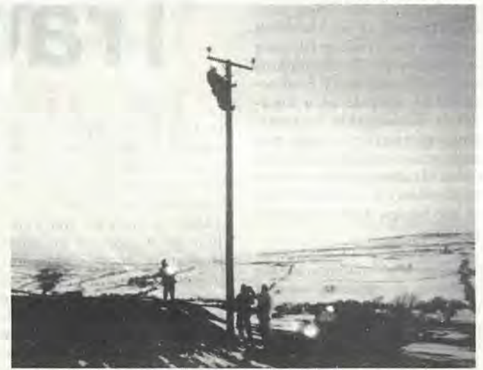
Dee Valley Apprentice Linesman Gary Clarke, at the top of the pole, and his colleagues work in darkness to repair an overhead line brought down in the heavy snow-fall at Cerrig.
